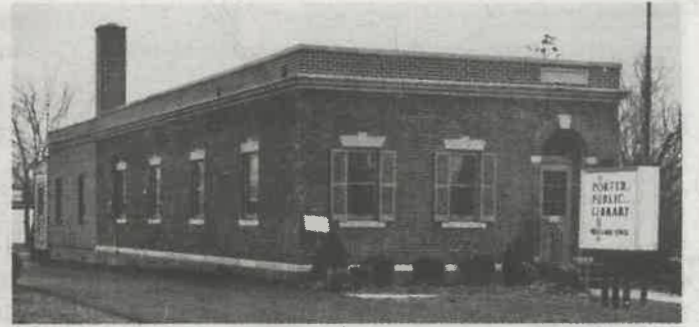
Westlake Porter Public Library in 1950 at 27059 Center Ridge Road.
